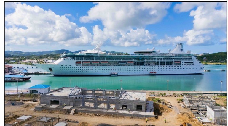
Upland Development In Progress as Cruise Terminal Advances
