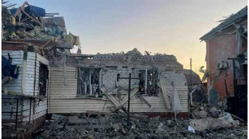
A damaged house following what Russian authorities called a Ukrainian military strike on the town of Sudzha.
