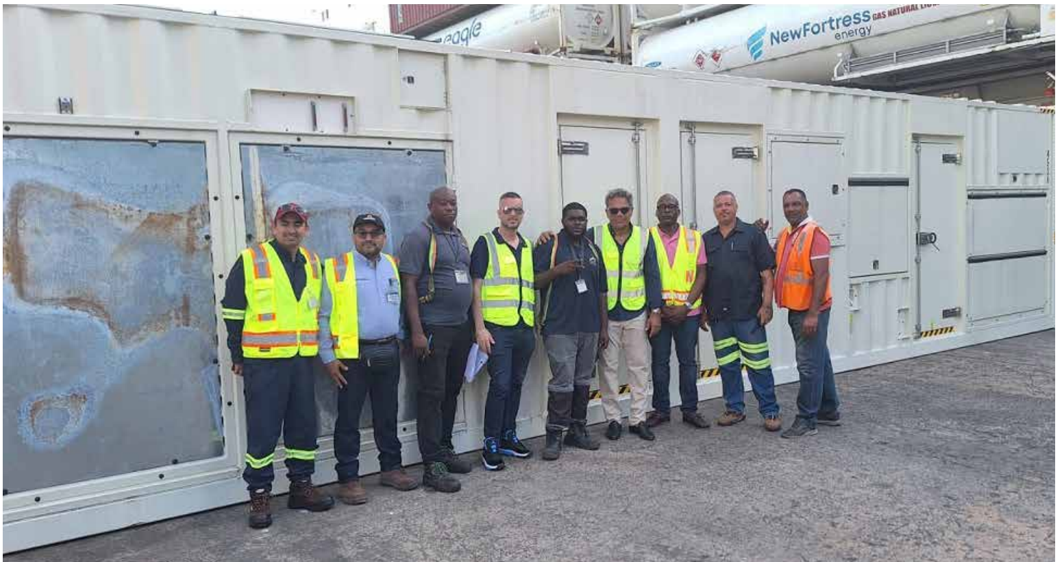
Arrival of Containerized Generators in Sint Maarten. (Photo credit: Government of Sint Maarten)
