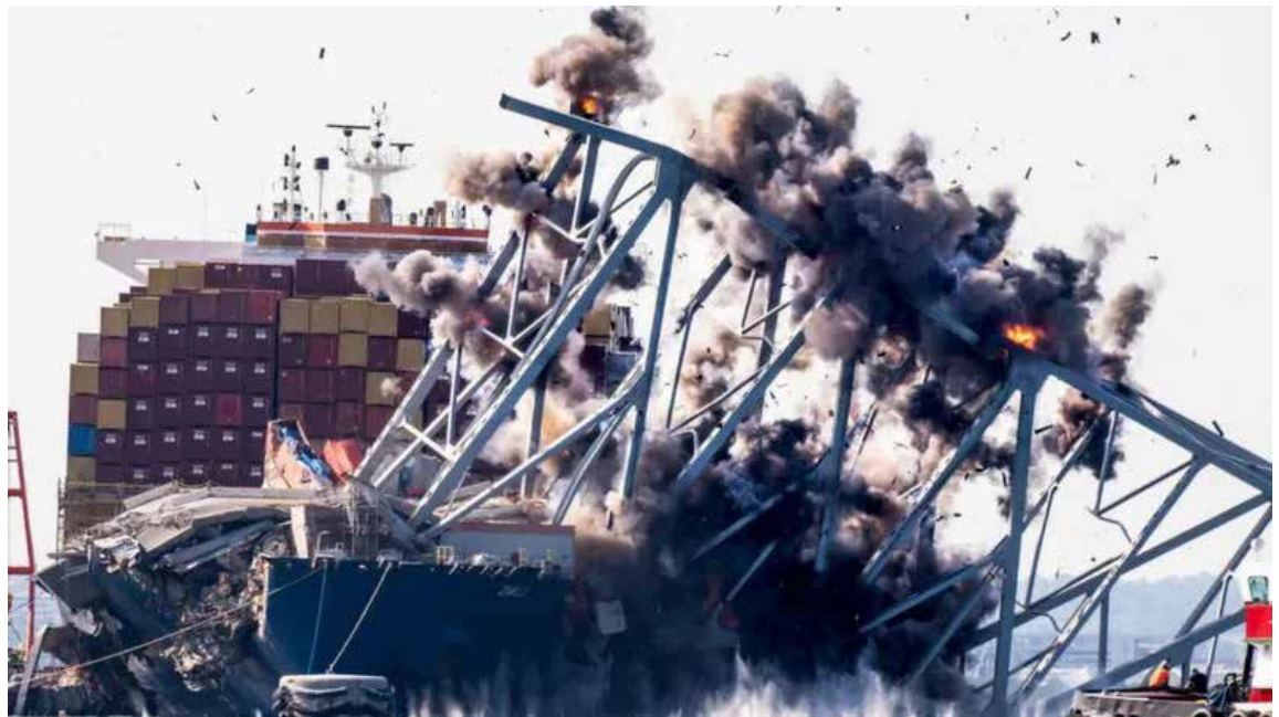
The crew of the Dali remained on-board even as explosives were used to destroy part of the Key Bridge on its hull.
