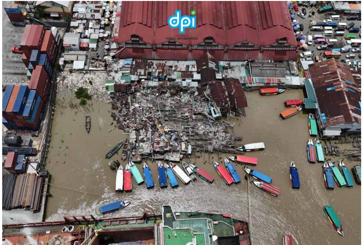
An aerial view of the collapsed section of the Stabroek Market. Photo: Department of Public Information.
