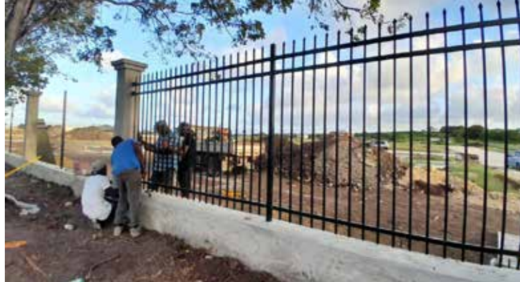
Work on fencing of the new cemetery at Tomlinson’s, as possible.
