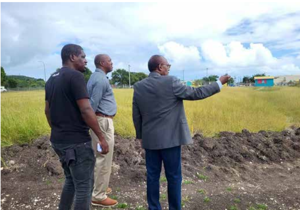
Road construction at the new Tomlinson's Cemetery
