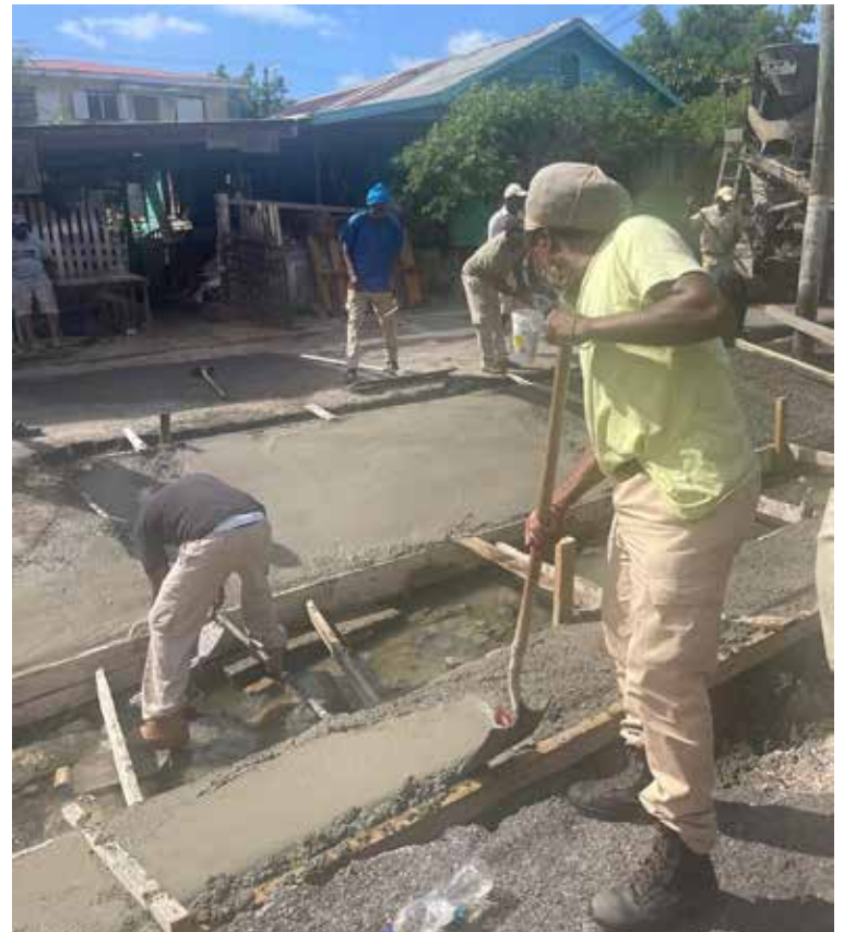
Work being done on Tanner Street.
