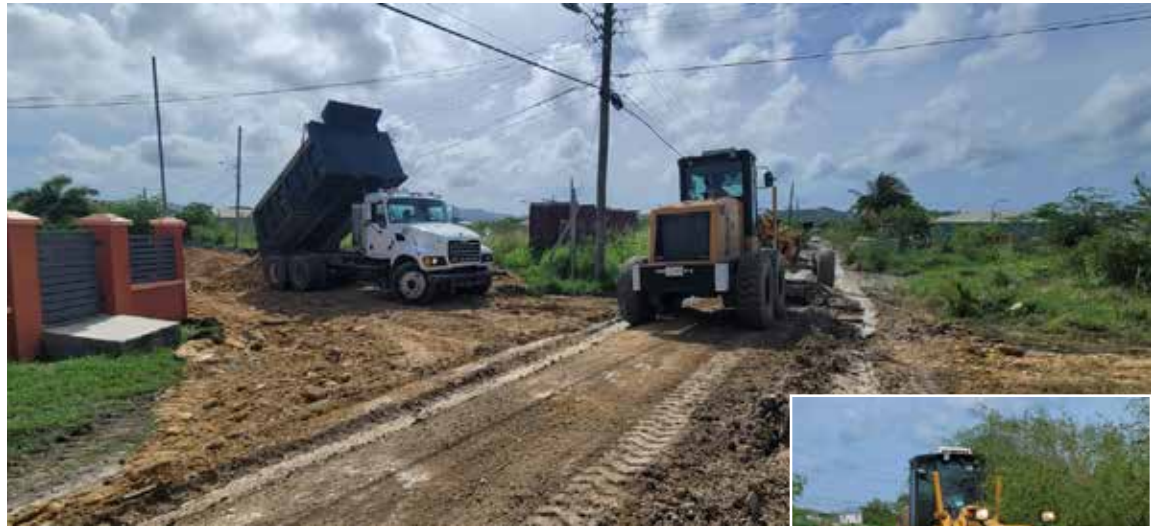
Heavy duty equipment at work in St. Peter.
