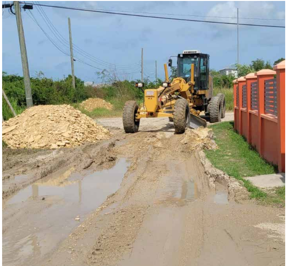
More work being done in St. Peter
