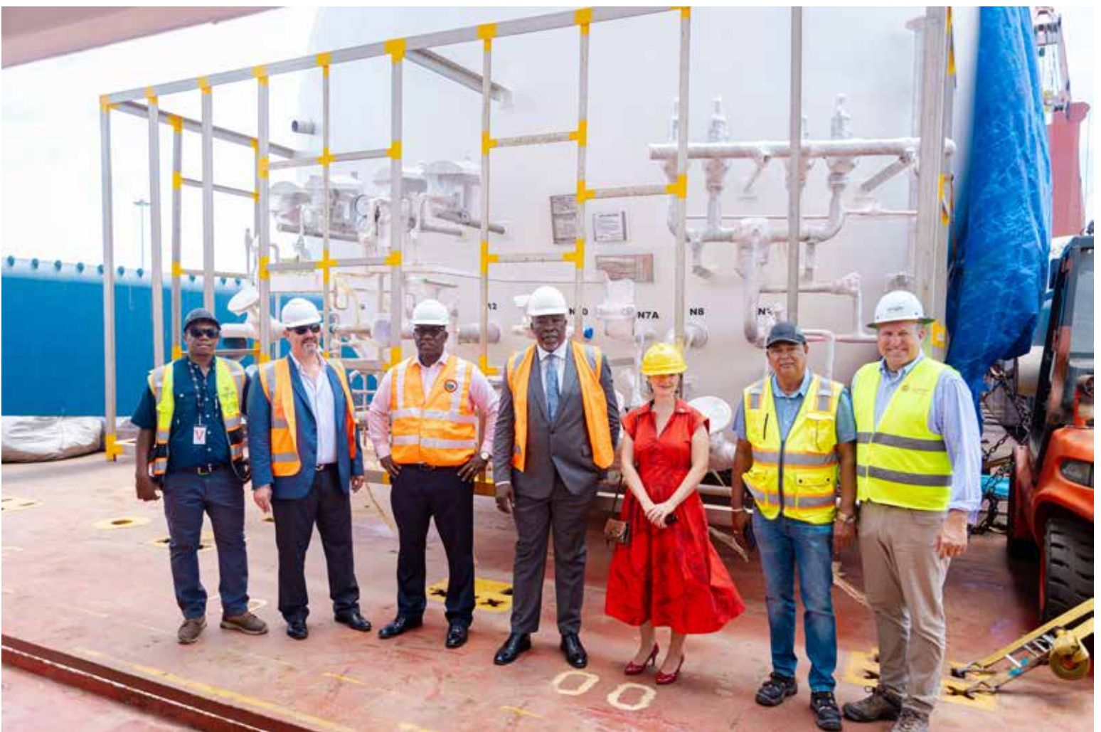
A team comprising representatives from the government, Antigua Power Company Ltd.-Caribbean LNG, and the US embassy in Barbados, were on hand to welcome the arrival of two huge storage tanks for the new Liquid Natural Gas (LNG) power plant being constructed at Crabbes. Story on page 4.
