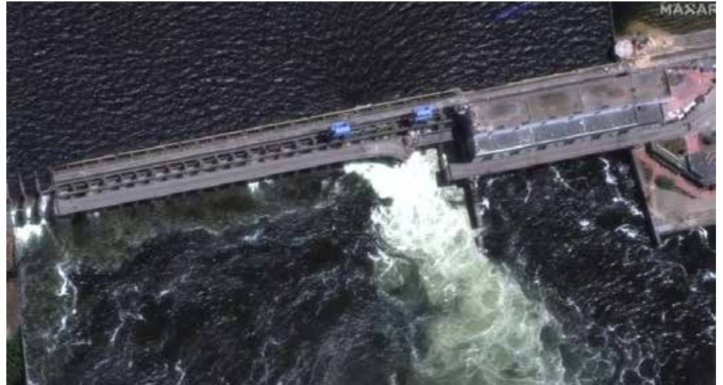
An aerial image shows water pouring through what appears to be a breach in the dam.
