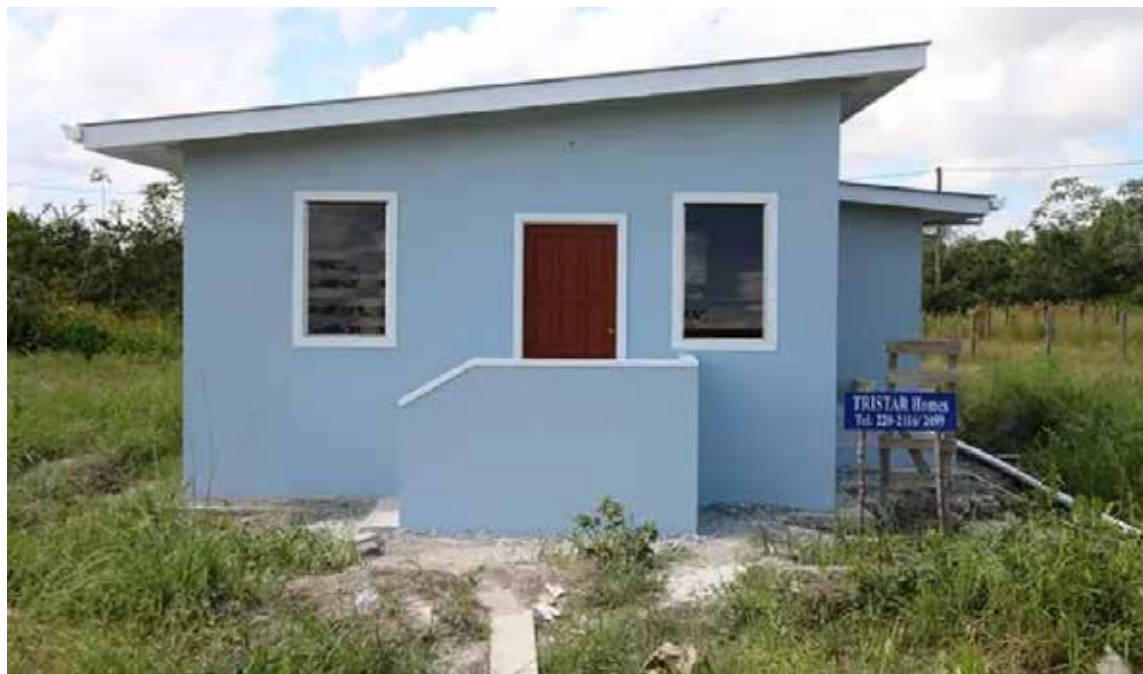
One of the cores constructed in Region Three. (Photo credit: DPI).
