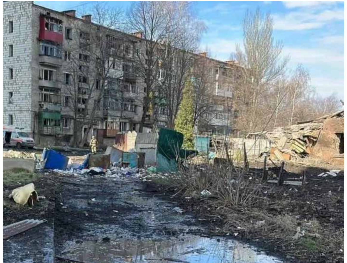
Ruined apartment blocks in Kostyantynivka.
