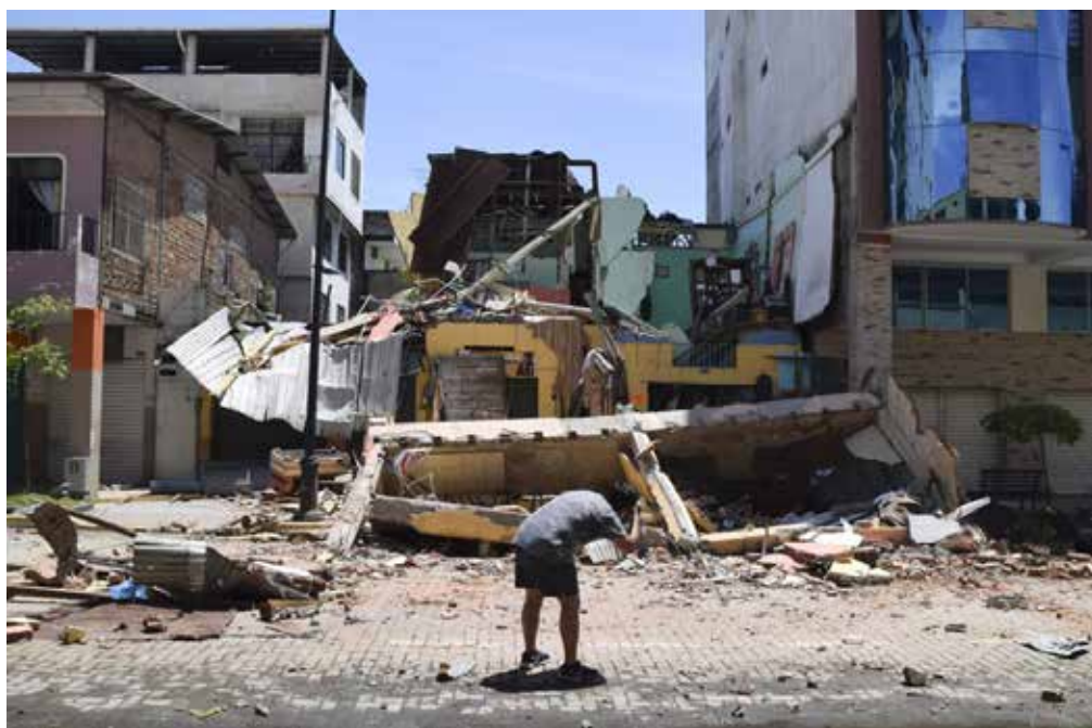
A man takes a photo of a building that collapsed after an earthquake shook Machala, Ecuador, Saturday, March 18, 2023. The U.S. Geological Survey reported an earthquake with a magnitude of about 6.8 that was centered just off the Pacific Coast, about 50 miles (80 kilometers) south of Guayaquil. (AP Photo/Jhonny Crespo)
