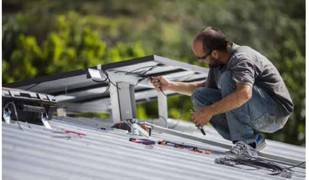
A technician installs a solar energy system at a home July 24, 2018, in Adjuntas, Puerto Rico. A U.S. government ongoing study that released preliminary results Monday, Jan. 23, 2023, has determined that with little room on the island for large-scale solar farms or wind generators, Puerto Rico should aim to reach its clean-energy goals by installing solar panels on all suitable rooftops, along with airports, brownfields and industrial areas. (AP Photo/Dennis M. Rivera Pichardo, File)
