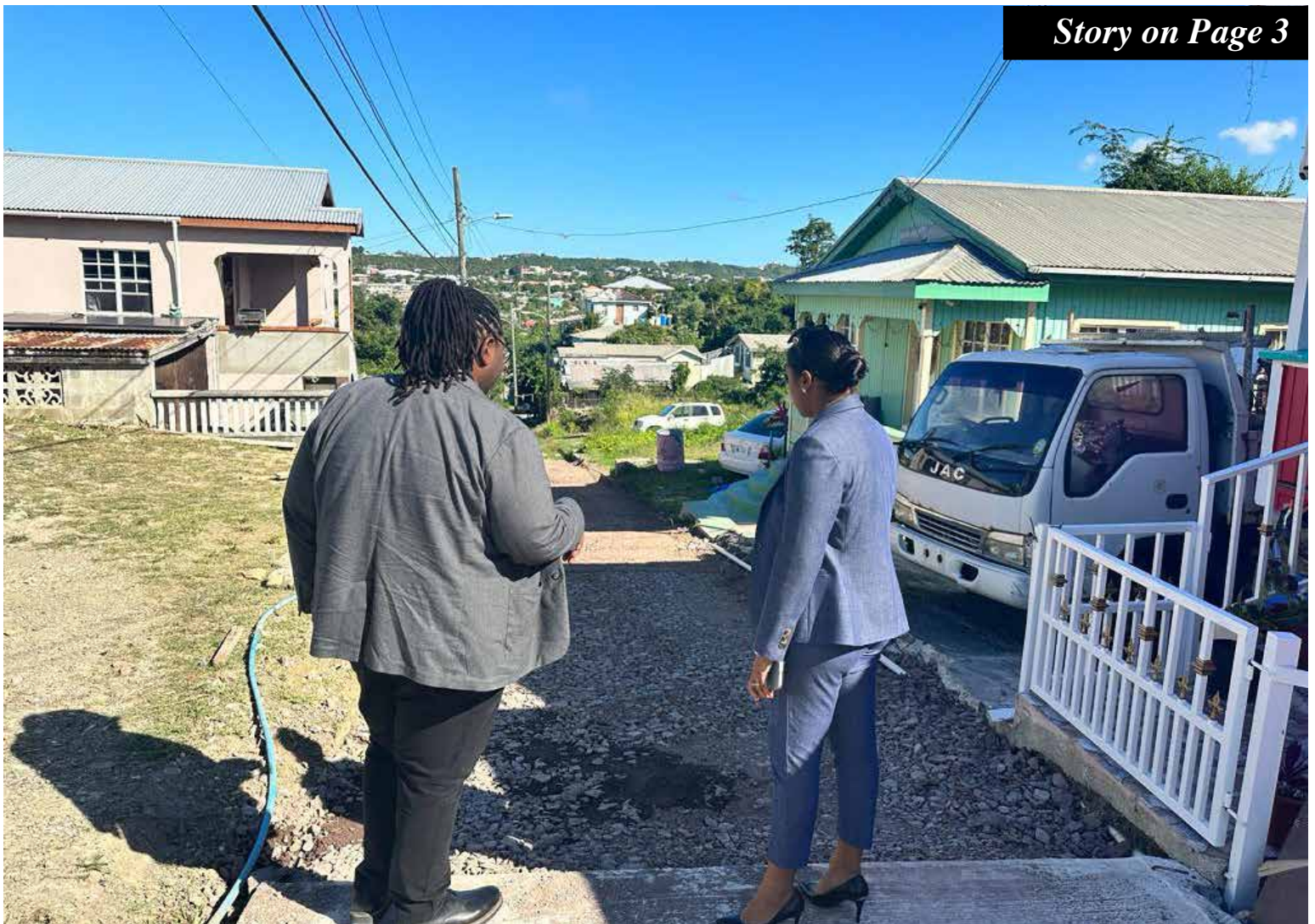
Works Minister Maria Browne (R) and Parliamentary Secretary Clement Antonio yesterday ordered the construction of a concrete road at Loblolly Street, Greenbay.
