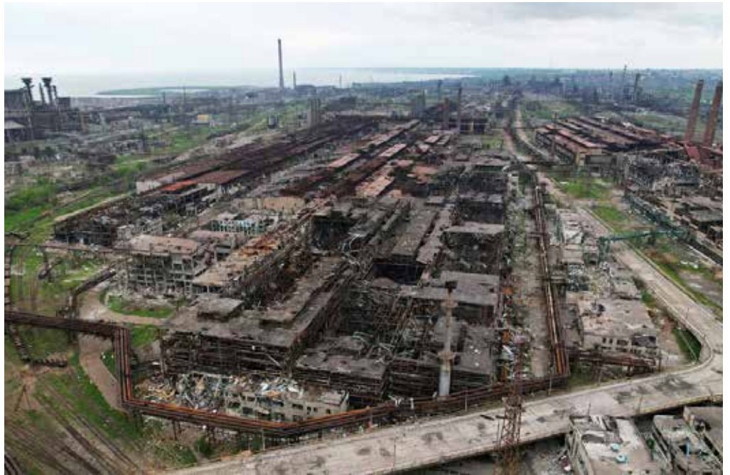
A view shows destroyed facilities of Azovstal Iron and Steel Works during Ukraine-Russia conflict in the southern port city of Mariupol, Ukraine May 22, 2022. Picture taken with a drone. REUTERS/Pavel Klimov
