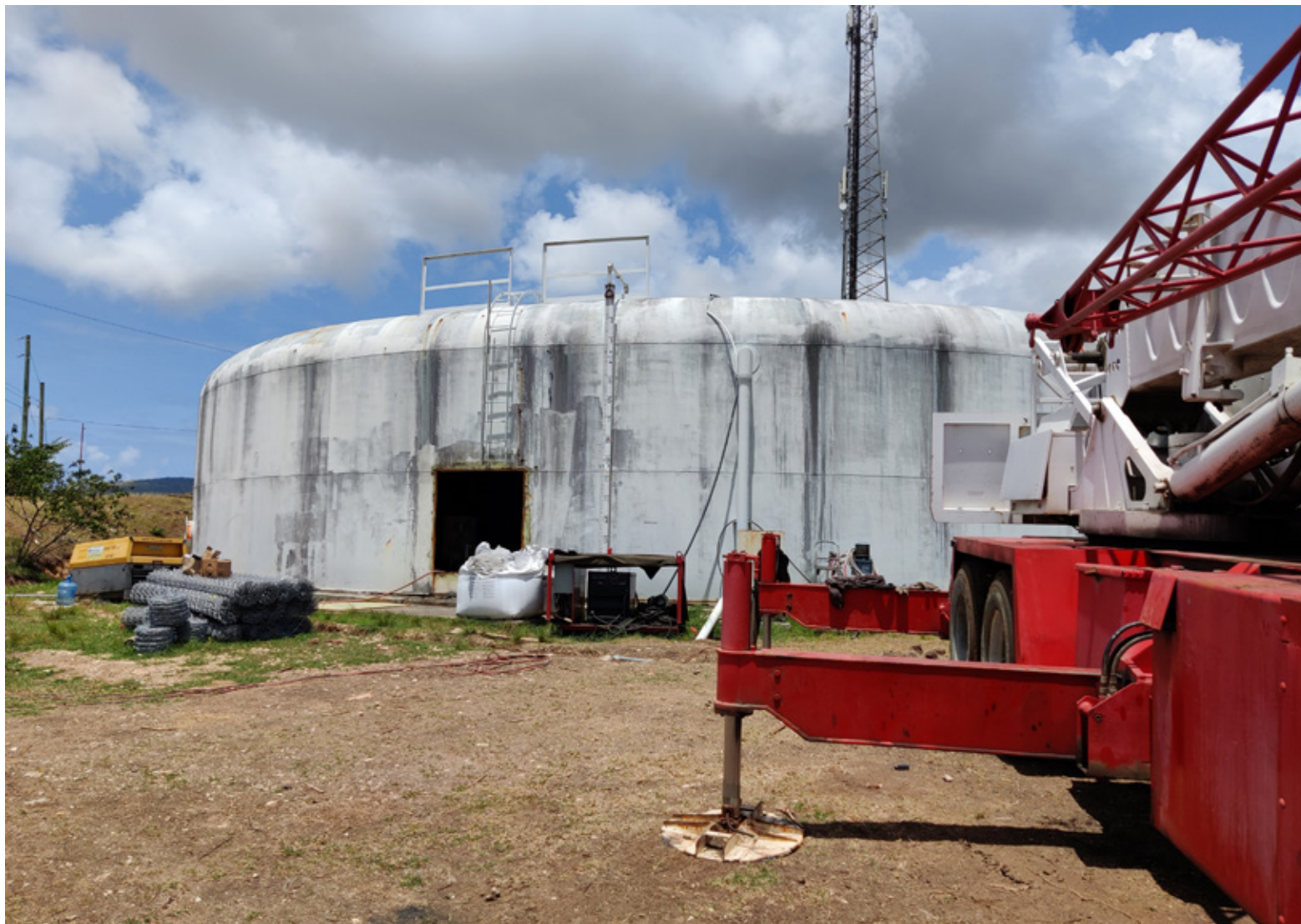
Disused potable water tank at All Saints being recommissioned.
