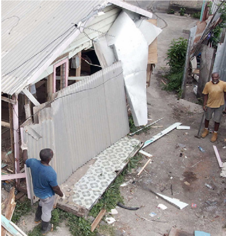
Photo caption: Demolition has started in the Booby Alley area.
