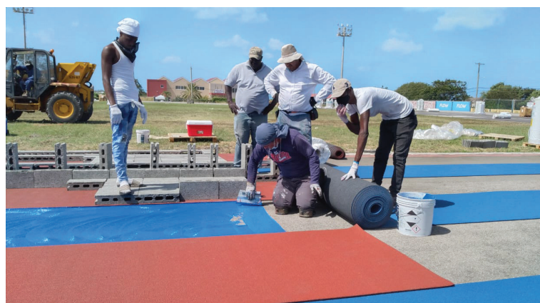
Laying of track at YASCO
